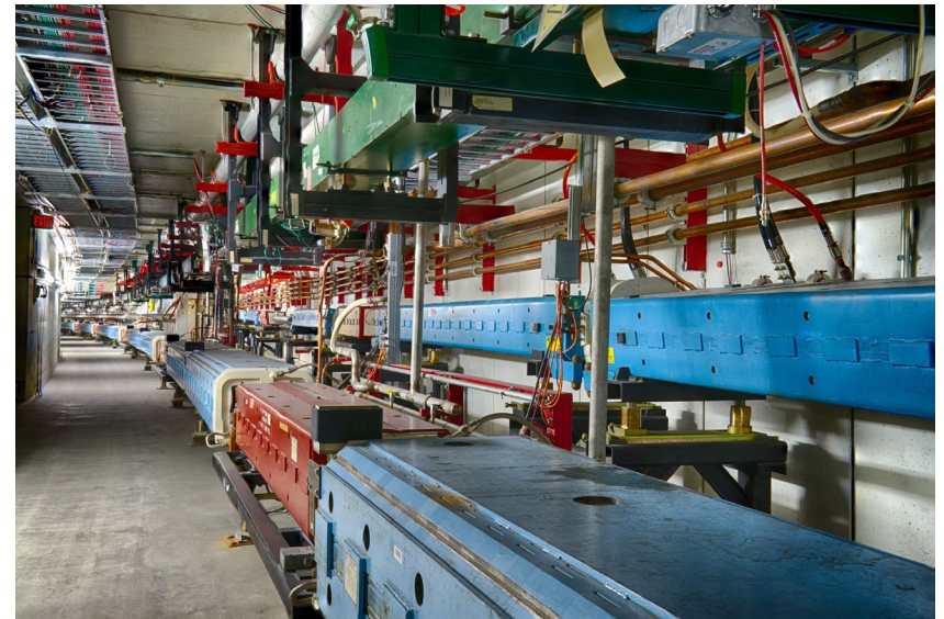
Fermilab Main Injector: Foundation of “Digital Twin” automation (2000)
